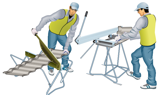
Fig 6.2.5.3 Hip tile being cut then bent
