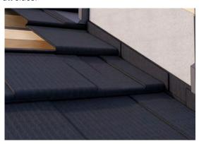
Prepare your back flashing. The head should have a 10mm turn-back to allow the next panel to hook into it.
