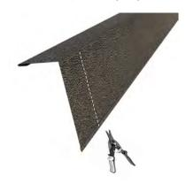
Make a horizontal cut to remove the bottom half of the newly-created flap.
