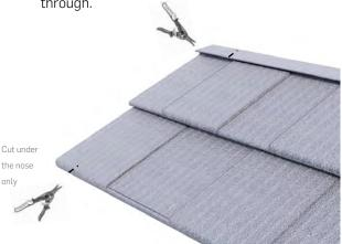
Then bend the side end of the panel to create a 40mm upstand. When installing the next course, add a bead of silicone to the join.
