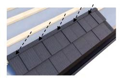
After installing the first panel, use the same method to fit the second panel over the first, overlapping at the weather channel. Push the panel upwards to secure in place, then fix with five fasteners.
