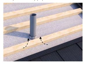
Install CF Shake or CF Shingle panels up the plane of the roof to the pipe. When the penetration is reached, pierce a hole in the panel at the centre of the pipe's location.
