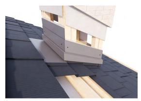
Once completed, the builders can install wall cladding to the chimney.
