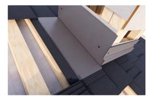
Finally, install a side flashing over the back flashing to align with the other already-installed side flashings.
